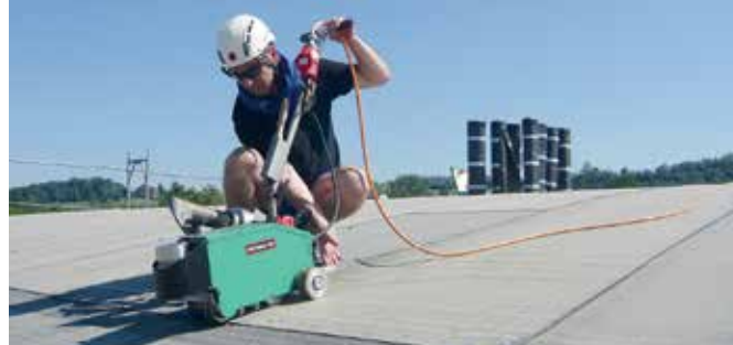
Flameless modified bitumen welding with the BITUMAT B2.
