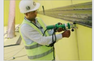
Waterstops welding in civil engineering
