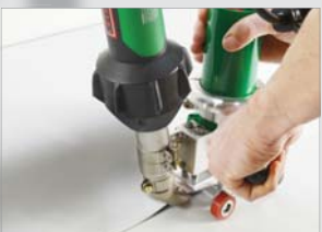
Welding close to the parapet
