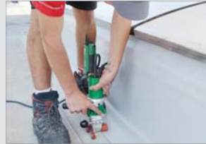
Welding close to the parapet at domed roof lights
